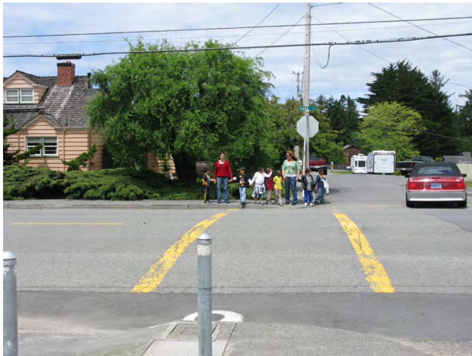
New ladder-style paint is needed to facilitate better visibility for the Park Street crosswalk in front of the school.
