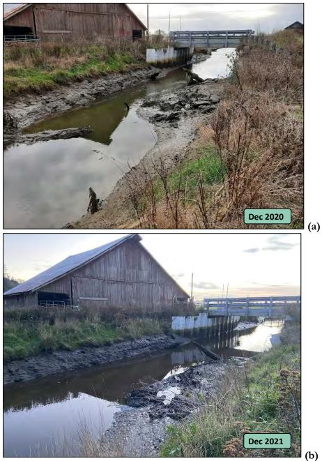
Figure 5. Bank slumping along the right side of the channel immediately upstream of the new bridge and sheet pile retaining wall, as seen (a) in December 2020 and (b) in December 2021 at low tide.
