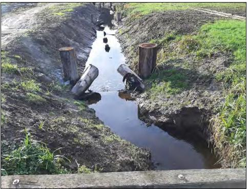
Figure 4. Upstream of the last weir where the project transitions back to the undisturbed channel. Alignment of the channel is creating some bank scour along the right bank.
