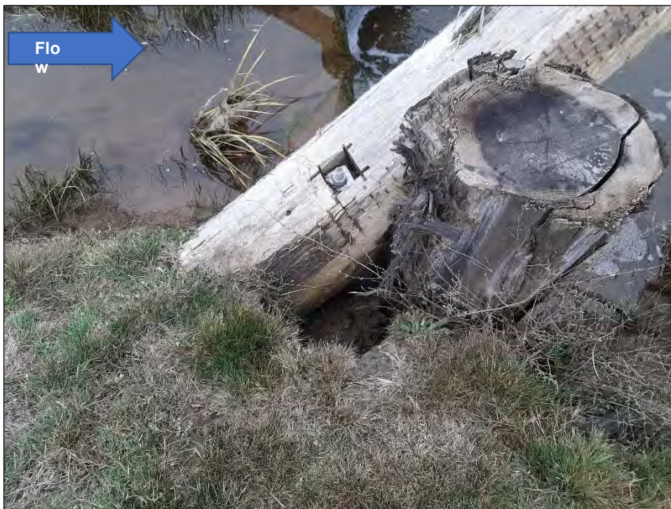
Figure 4. On December 22, 2019 (a) high flows overtopped the banks at Pond D and the channel draining the pond into Martin Slough, causing flow to flank the log weirs and (b) causing scour pockets behind the training logs located on top of the weir logs.
