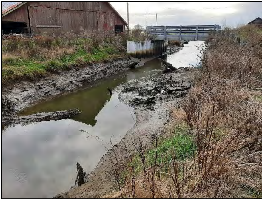
Figure 3. Bank slumping along the right side of the channel immediately upstream of the new bridge and sheet pile retaining wall, as seen (a) in December 2019 and (b) in December 2020 at low tide.
