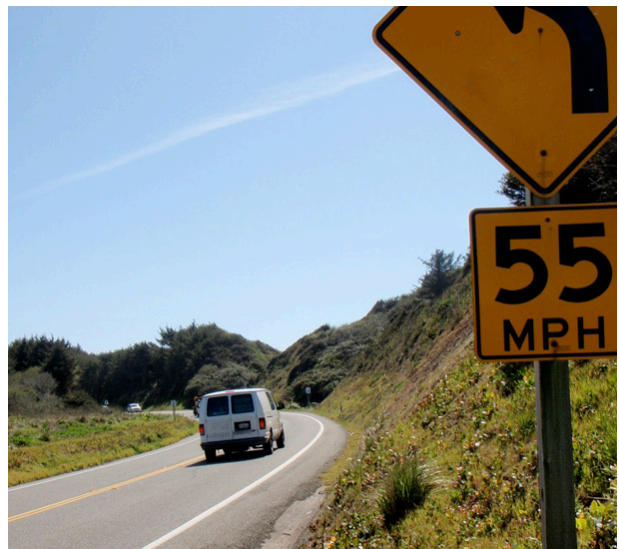
The US 101 corridor at Gyon Bluffs experiences high vehicle speeds and is very narrow with limited sight distance
