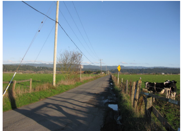
Roadways such as Miller Lane, pictured above, are narrow and constrained by ROW, fences, drainage ditches and utilities.
